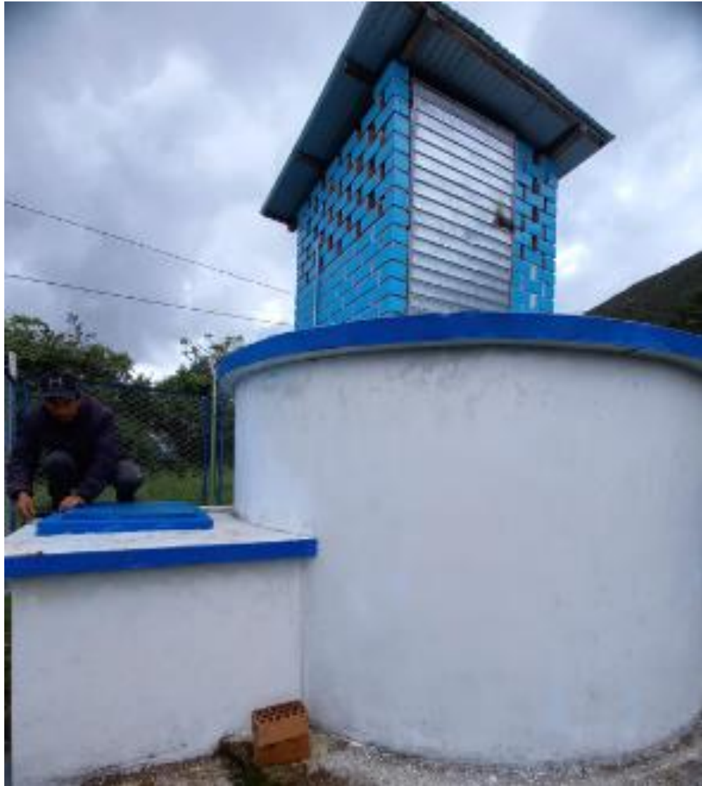
Reservorio N°1 circular 13m 3
